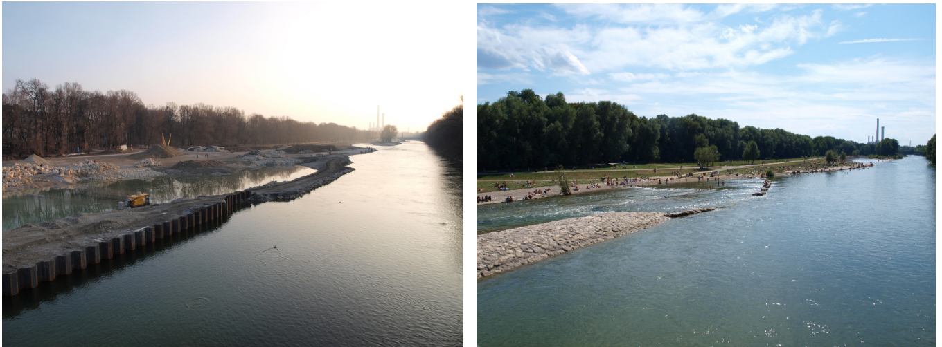
Figure 2.8 The Isar river during (left) and after (right) the hydro-morphological restoration. Today's near-natural landscape raises awareness on the usefulness of NBSs both for DRR and recreational purposes (Pictures: Zingraff-Hamed 2011 and 2015).
